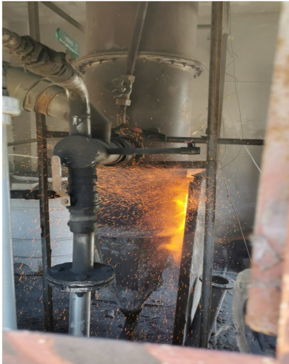
Figure 5. The biomass-oil shale burner.
