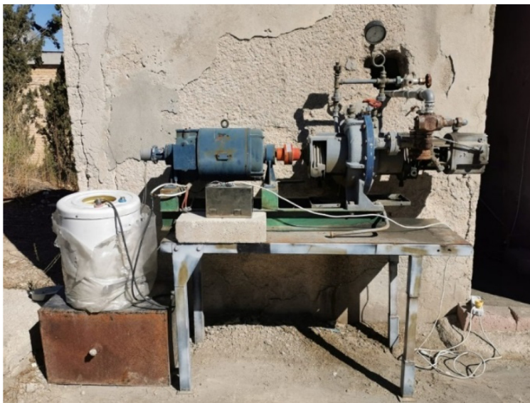
Figure 7. The coupled steam turbine and generator.
